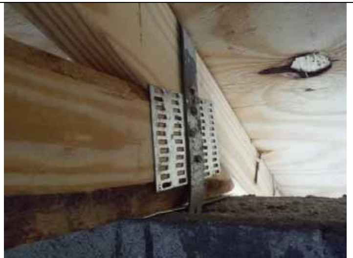
Roof to wall attachment
