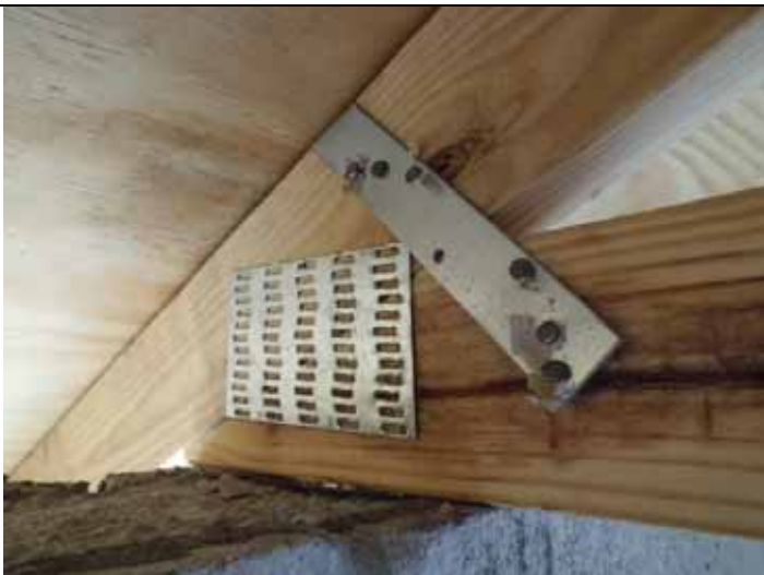
Roof to wall attachment
